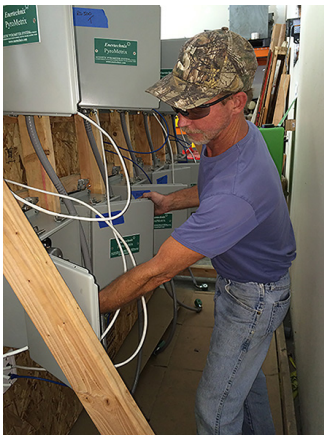
Enertech Staff Installing Clean Technology Sensors
