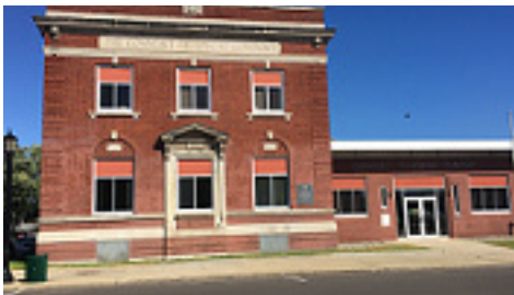
GreatWave Broadband Services Building
