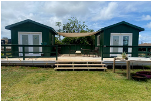
Two Completed Ohana Units
