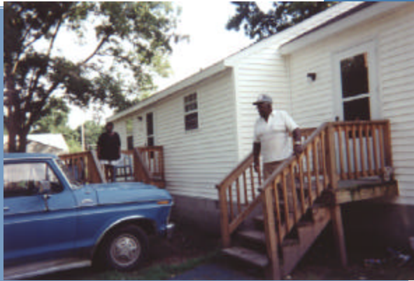
The New Road Community Development Group has renovated several homes like this one for the residents of its community. New Road receives technical assistance from the Virginia Eastern Shore Economic Empowerment and Housing Corp., funded by Rural LISC, a CDFI Fund awardee.
